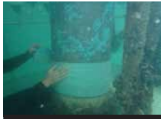
EXTERNAL CRACKS IN EXISTING SYSTEM AND SPREAD OF CORROSION UNDER FILM
