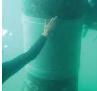
APPLICATION OF STOPAQ WRAPPINGBAND SZ
