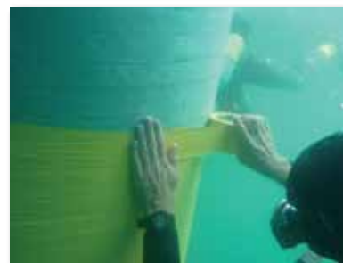
APPLICATION OF INTERMEDIATE LAYER / PVC YELLOW AND OUTERGLASS XT 24
