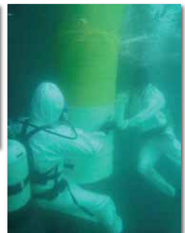
APPLICATION OF INTERMEDIATE LAYER / PVC YELLOW AND OUTERGLASS XT 24
